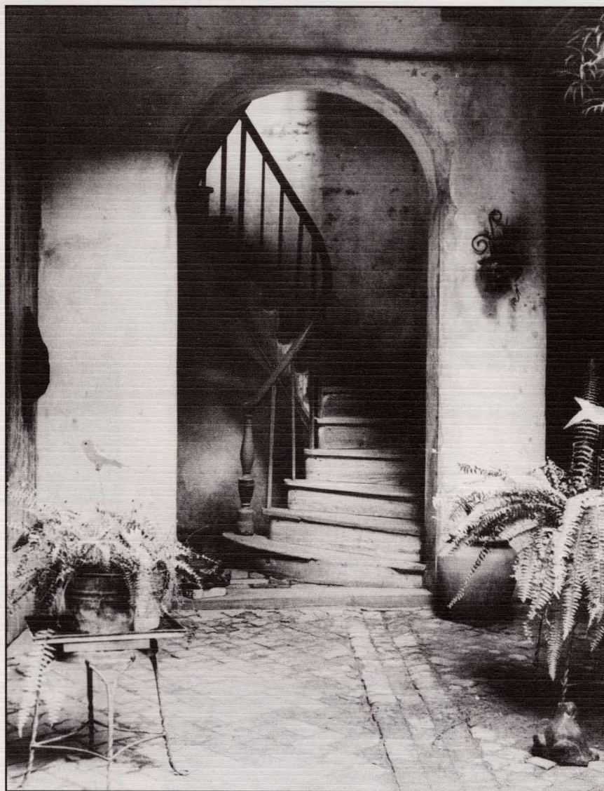
Marchand Patio and Stair, 830 Royal Street (1978.102.73.1)
