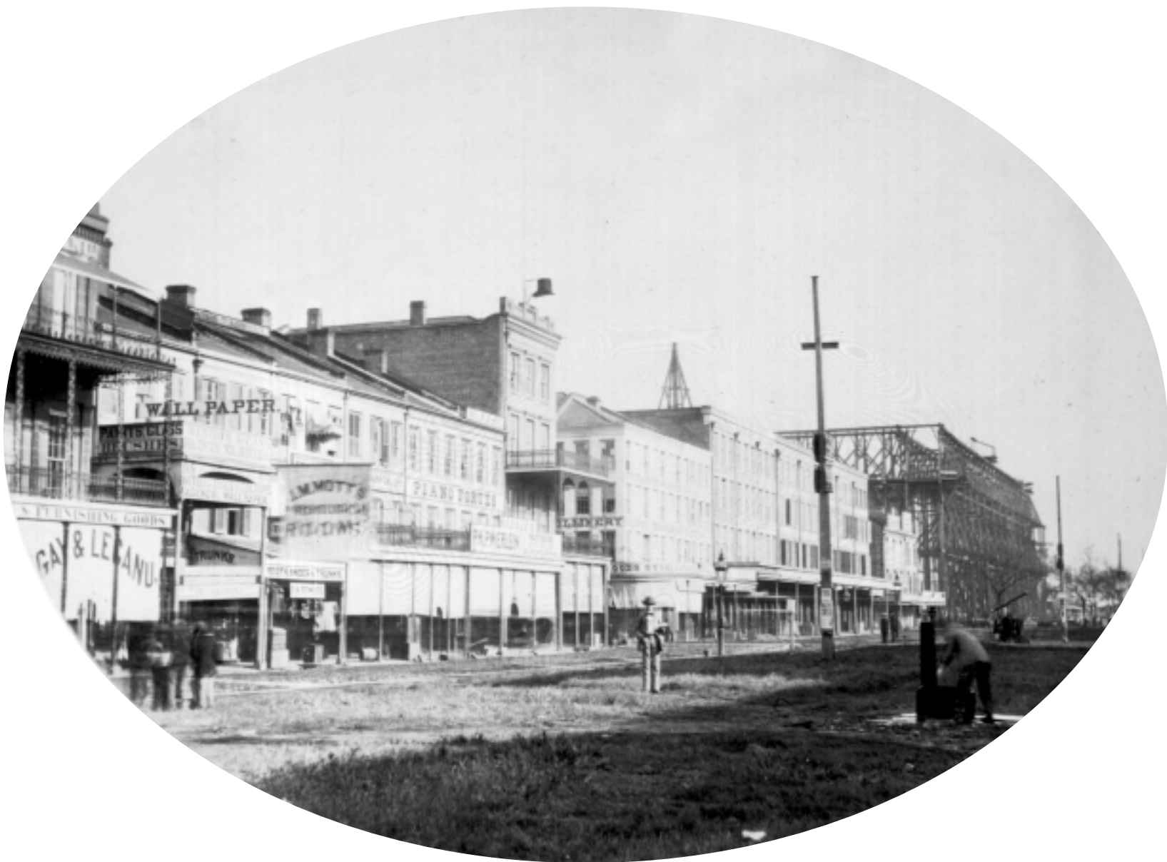
North side of Canal Street, 400-600 blocks, showing the Custom House under construction, surrounded by scaffolding, Jay Dearborn Edwards, photographer; between 1857 and 1860 (1982.32.2).
